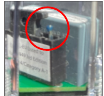
Expended Condition: Blue flag not under hood
