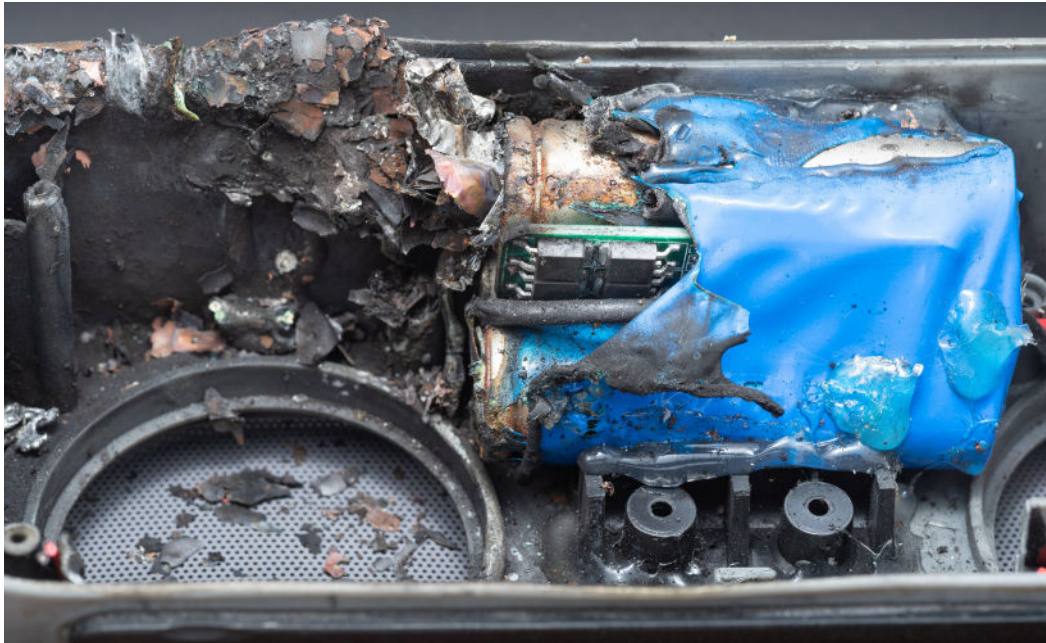
Image 2: Heat-damaged Lithium-ion Battery
