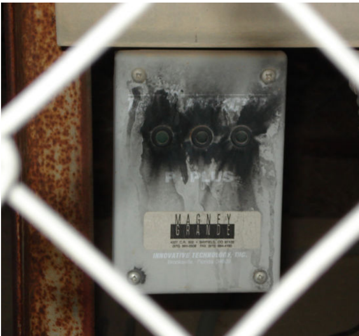
Image 2 Catastrophic SPD Failures
